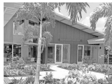
The new Shelly Stayer Shelter is 22,500 square feet and has 60 total beds. COURTESY OF THE SHELTER FOR ABUSED WOMEN AND CHILDREN
